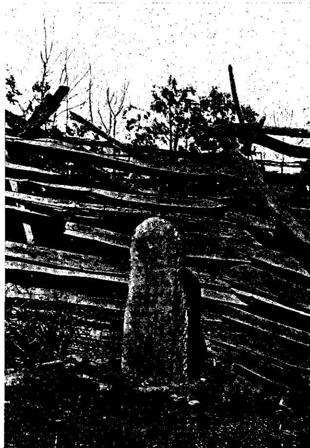
FIG. 2.—MONUMENT (NO. 223) ERECTED IN 1860 BY LT. MICHLER AT NORTH END OF MICHLER LINE TO MARK NORTHWEST CORNER OF MARYLAND. NOT ACCEPTED BY MARYLAND.
